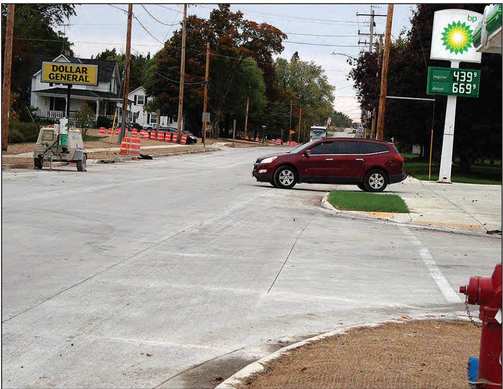
The stretch of Highway 22 going through Gillett is pretty much done, except for striping and a few minor things. The city will be holding a ribbon cutting ceremony Oct. 16 to celebrate the completion of the year-long project.
