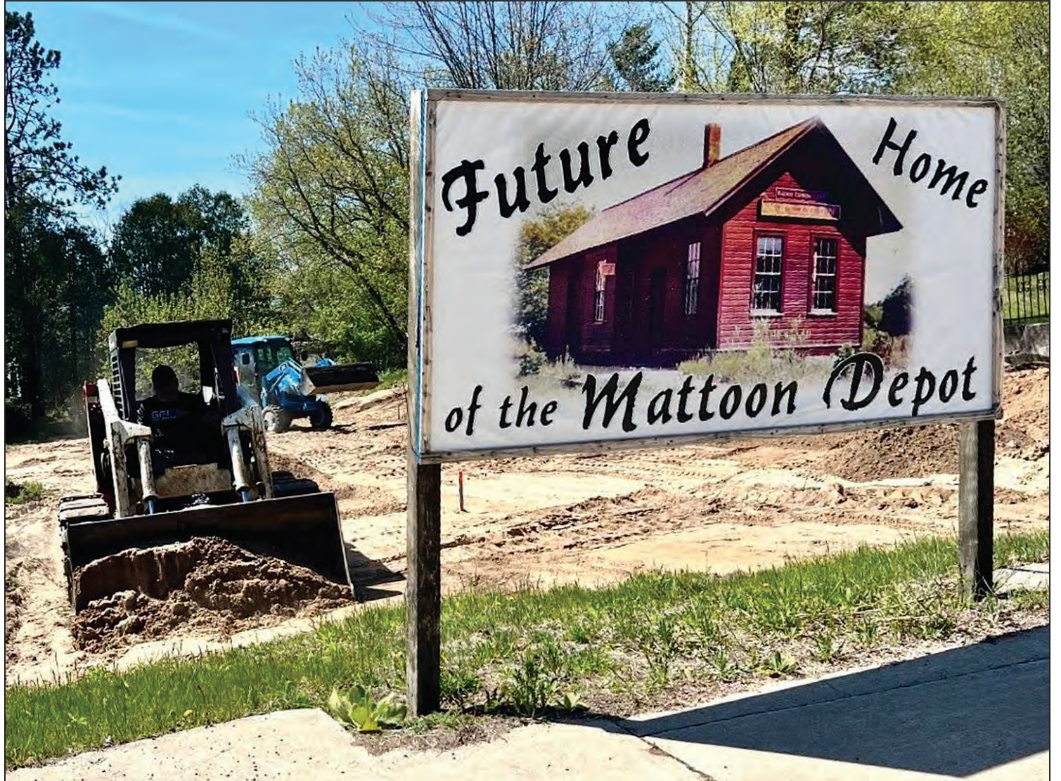
The construction of Mattoon's historical train depot replica is coming along. Excavation was completed in May and June by Jess White and Dave Kickhaver, both original members of the Mattoon Area Historical Society.
