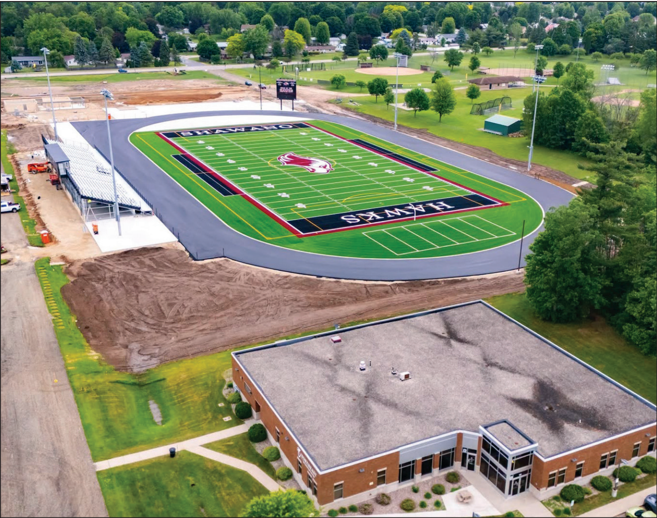
Shawano Community High School's new stadium, part of a $51.23 referendum approved by voters in November 2024, will feature an upgraded eight-lane running track circling the football and soccer field, new grandstands with built-in storage spaces underneath, a dedicated and updated tracking and throwing areas for field events, expanded gathering spaces, updated restrooms, redesigned traffic flow, a new ticket booth and a new concession stand.
