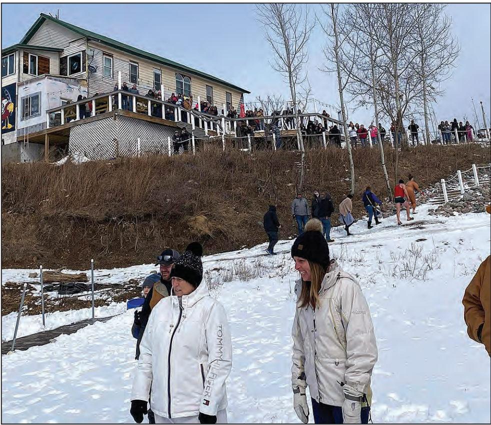
Little Tippy is the oldest commercial building in Townsend and one of the funner places in the town, but a catastrophic water leak has closed the original Wheeler Hotel while repairs are made, impacting the building's summer revenue potential.
