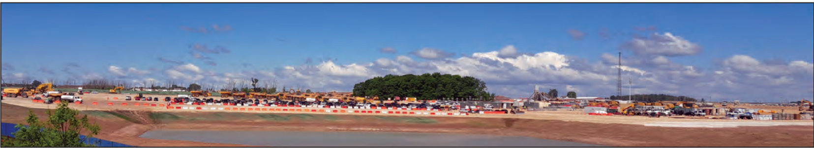
The Port Washington data center is a $15 billion-plus artificial intelligence campus under construction by Vantage Data Centers. Known as the Lighthouse campus, the 672-acre site will host four centers spanning 2.5 million square feet with almost 1 gigawatt of IT capacity, creating up to 4,000 construction jobs and 300-plus permanent positions.
