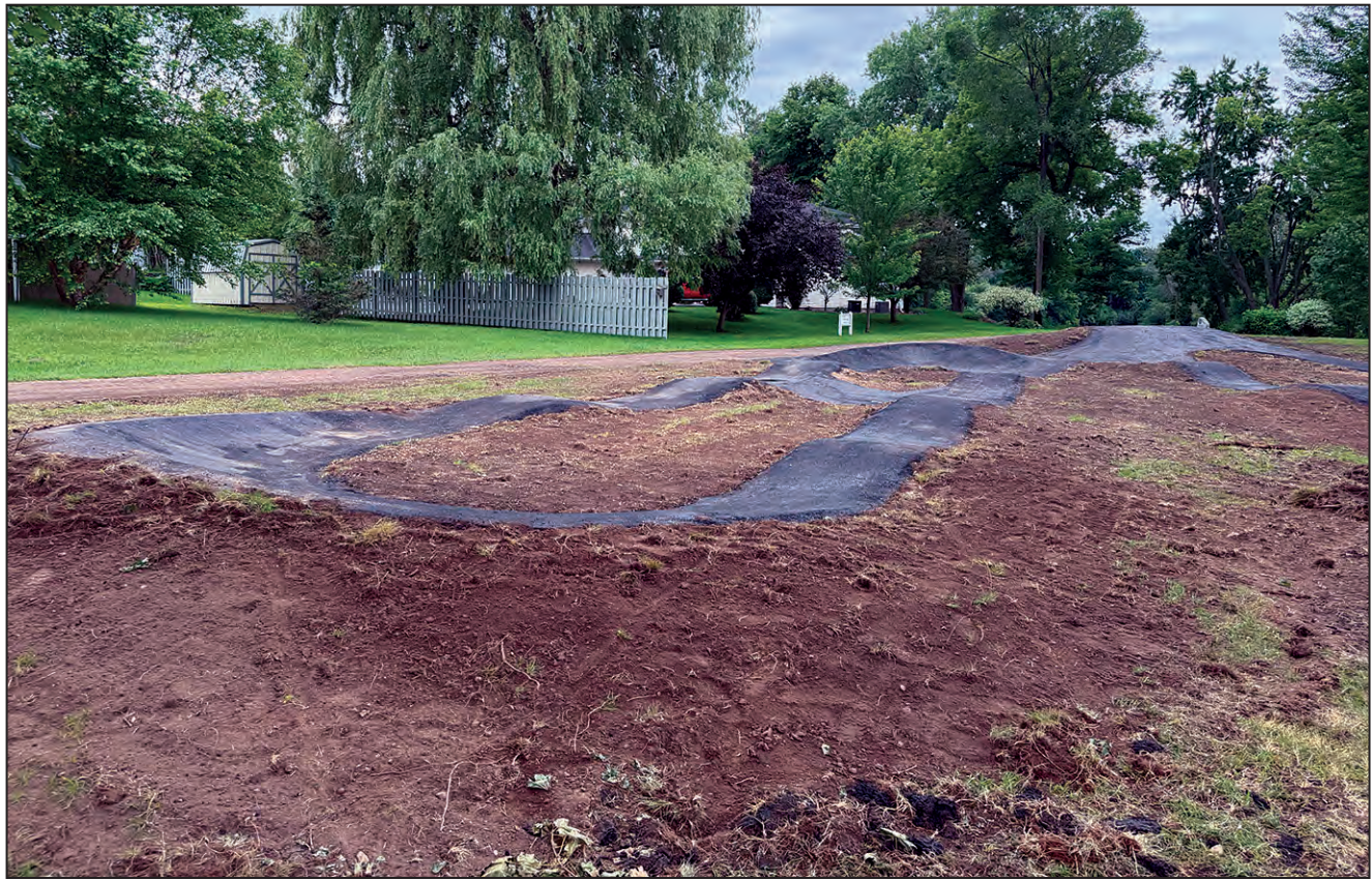
Pictured while still under construction, the new pump track at Kuckuk Park is open and ready for use. The track features two connected tracks, one beginner and one intermediate, designed to create a continuous loop with the existing pathway. Riders build momentum while navigating small features and jumps.
