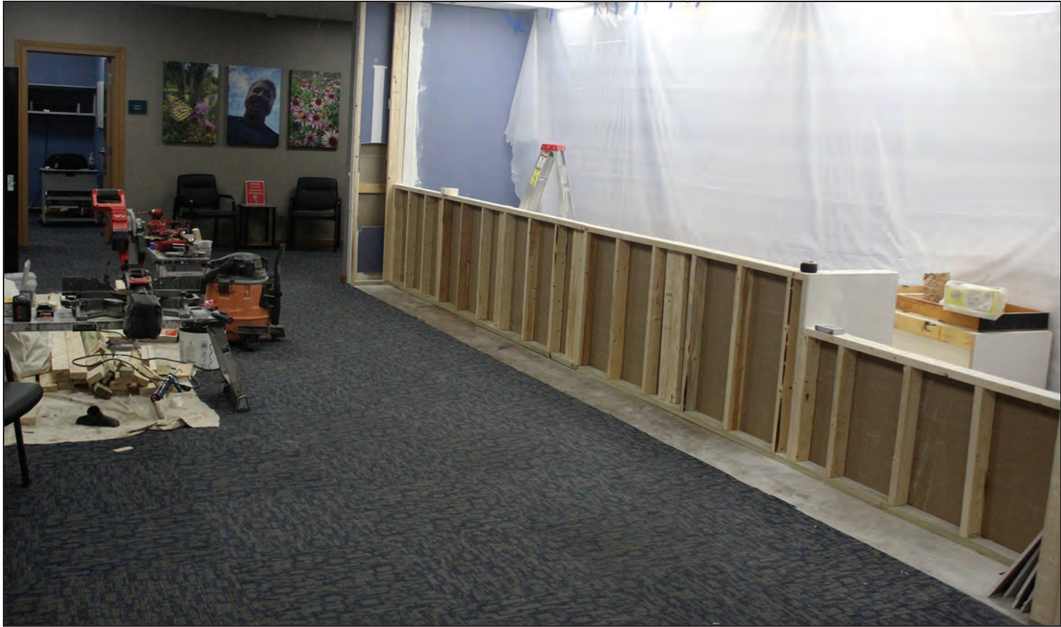
Work is currently being done on the reception area at Shawano City Hall with new counters, safety glass and more going in. The work is expected to be completed the first week of March.
