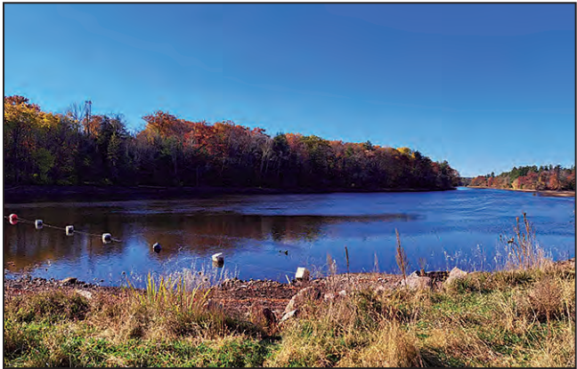
The Wolf River north of the Balsam Row Road Dam is lower than normal as Wolf River Hydro LP officials continue their project to repair the dam's gate seals. The drawdown is expected to end when it reaches 9 feet.
