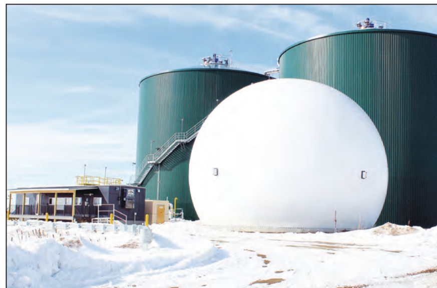
Tanks and snow sit on the DTE Vantage facility near Matsche Farms, Inc. in Birnamwood. The biomass processing plant opened last month, taking waste from Matsche cattle and turning it into natural gas for use in vehicles in California.
