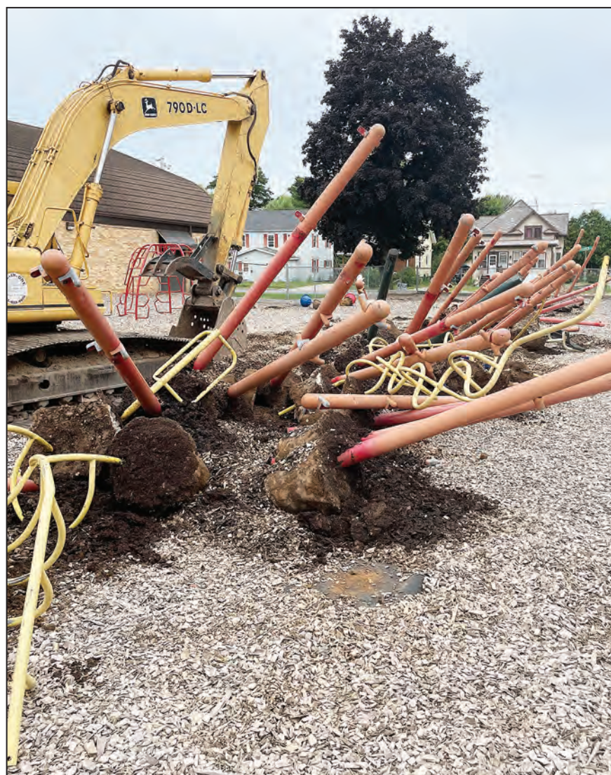
Old playground equipment is being removed outside St. James Lutheran School to make way for new equipment, paid for by fundraisers and grants. CONTRIBUTED
