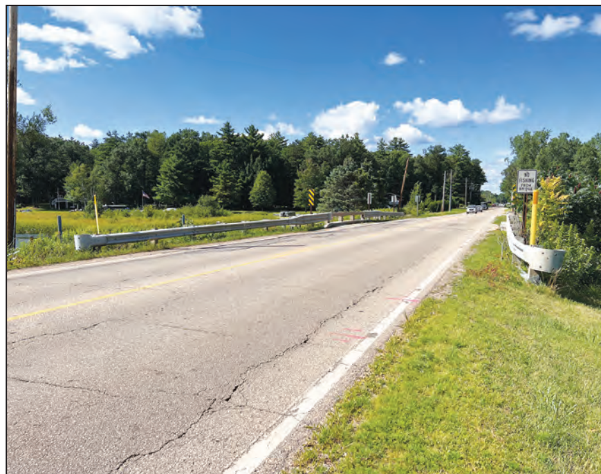
The bridge on County Road HHH is set to start being replaced on Aug. 8. Construction on the bridge will continue through the first week of November. The bridge is being replaced in order for upgrades and to add more room for boating, walking and snowmobiling traffic.
