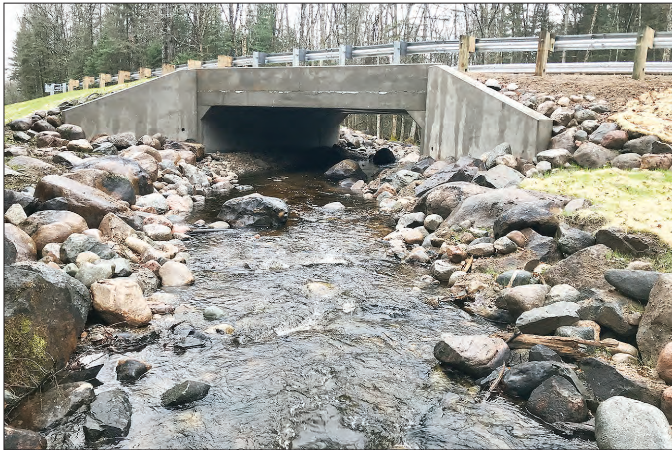
Trout Unlimited worked with the U.S. Forest Service on a trout habitat improvement project on Rock Creek, a tributary of the Peshtigo River in Forest County. TROUT UNLIMITED
