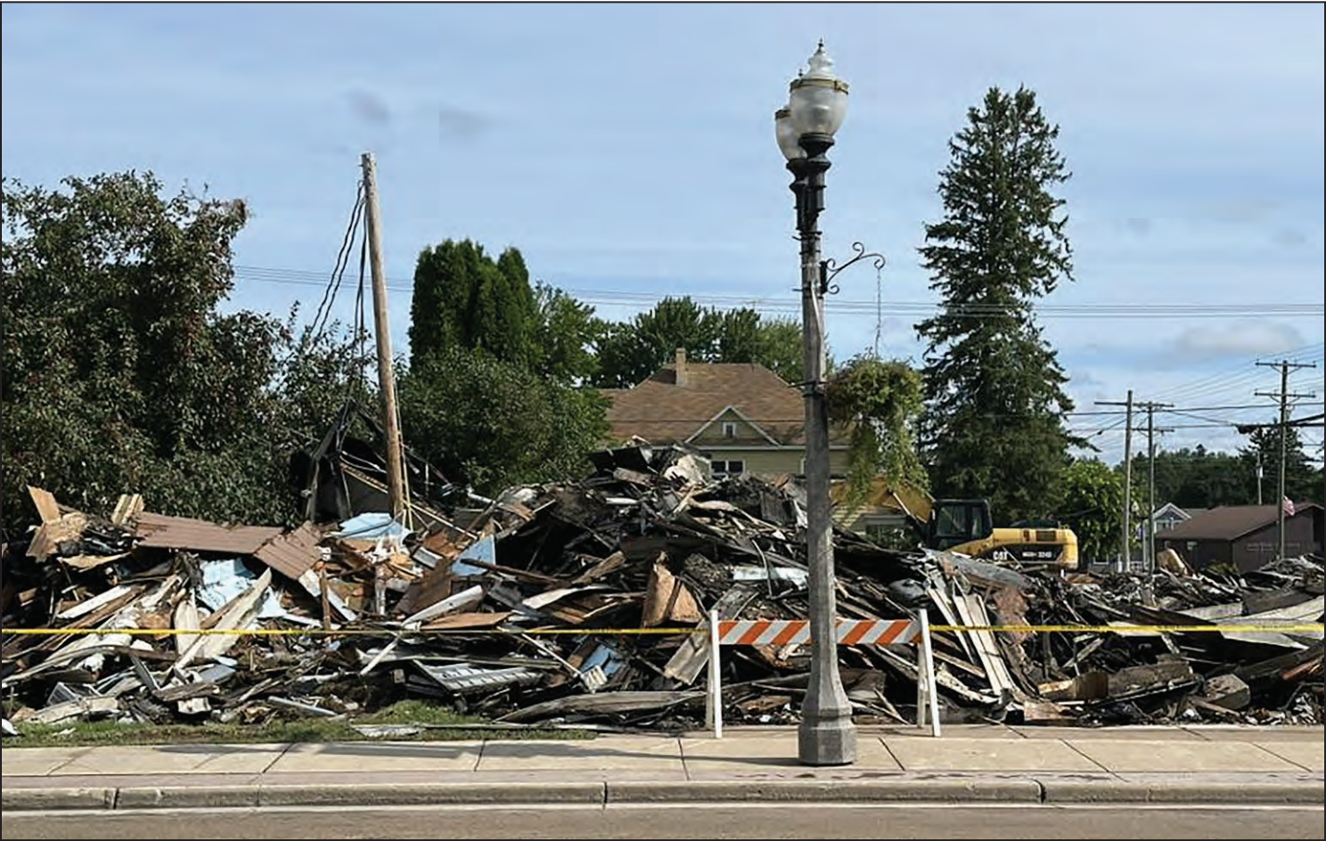
The remains of an Aug. 16 fire can be seen in downtown Tigerton the day after the blaze destroyed a business and apartments. Three families are now in need of clothing and household items.
