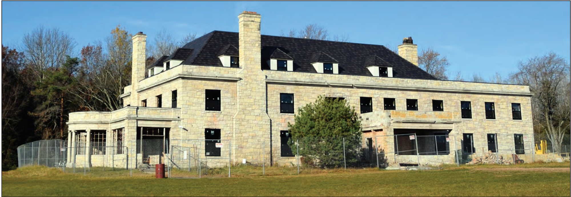
All that remains of the former Alexian Brothers Novitiate complex is the original mansion built in 1939. A 2022 restoration project included gutting the interior and installing a new roof and windows. Owners Ethan and Stephanie Fernhaber are working to bring new life to the 25,827-square-foot mansion that rests on the 177 acres along the Red River. CONTRIBUTED
