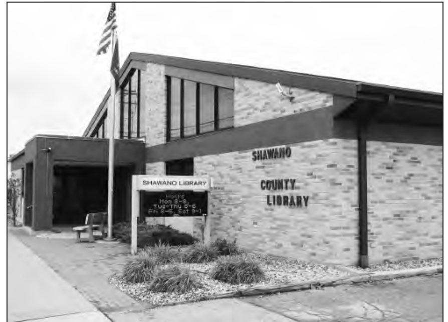
Water leaks and severe mold issues may force the early closure of the Shawano County Library, county supervisors were warned Sept. 27. The library board is expected to discuss the issue and possible temporary relocation to an alternate site.
