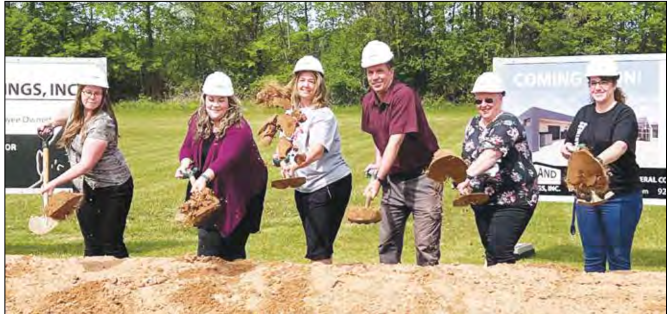
Members of the Bowler school administration — led by Superintendent Glenda Butterfield-Boldig, third from left — throw dirt in the air to celebrate the groundbreaking of the new Bowler agriculture and technology building on May 31. The building will be home to a greenhouse class, an aquaponics class and animals that students will raise for the Shawano County Fair.
