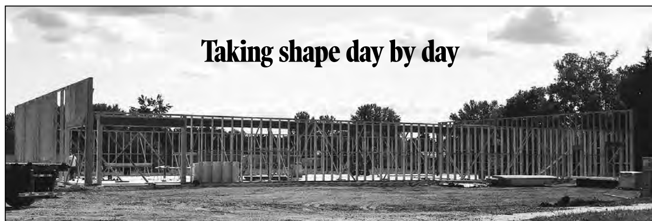
Crews have the frame of the new Dollar General store in place at the corner of McKenzie Avenue and Park Street in the City of Gillett. The store is expected to open by the end of the year.
