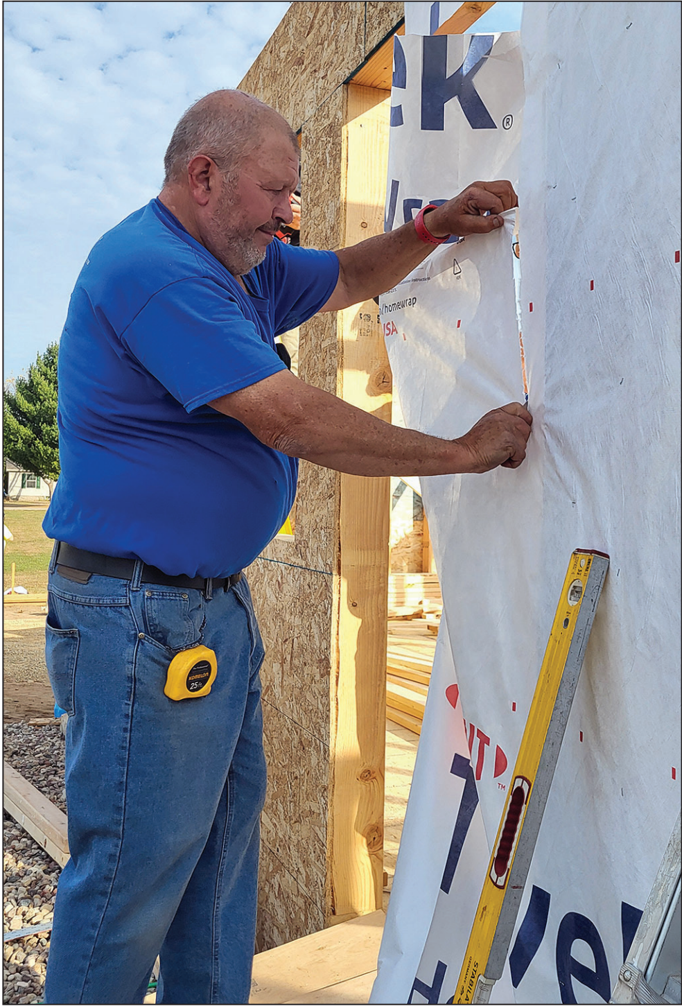
Mark Flunker attaches Tyvek HomeWrap to a new home being built by Wolf River Habitat for Humanity in Gresham on one of his last days as construction supervisor for the Shawano-based housing ministry. Flunker retired on Nov. 2 after 10 years with the organization. The Gresham home is being built for a couple with three children, who are investing 500 of their own sweat equity into the property.
