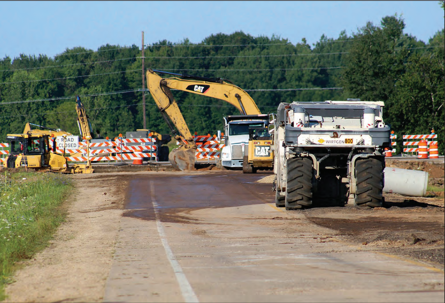
The second of four phases for the reconstruction of the intersection of state Highway 29 and County Road MMM is underway. This phase began July 22 and will last a total of five to seven weeks. The intersection is completely closed to through traffic.
