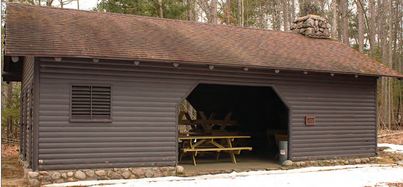
A historic shelter in Mountain's Green Lake Park is scheduled for some major renovations this year. The Civilian Conservation Corps built the shelter in 1937. GREG SEUBERT
