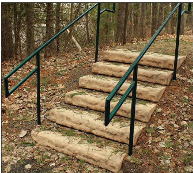
A new set of stairs and railing leading to the boat landing is one of the recent improvements to Green Lake Park. GREG SEUBERT
