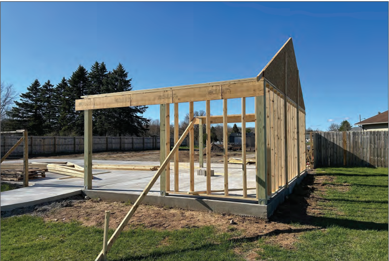
The bones of the new pavilion at the Oconto Falls Community Garden can be seen May 3. The structure is expected to be used for educational programs and other events at the garden.
