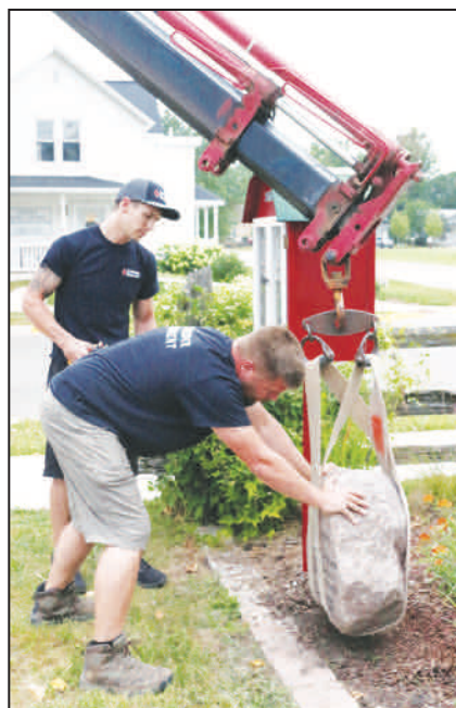
Schneider Monument's Chad Spaeth sets the memorial stone in place with help from Matt Kretschmann.
