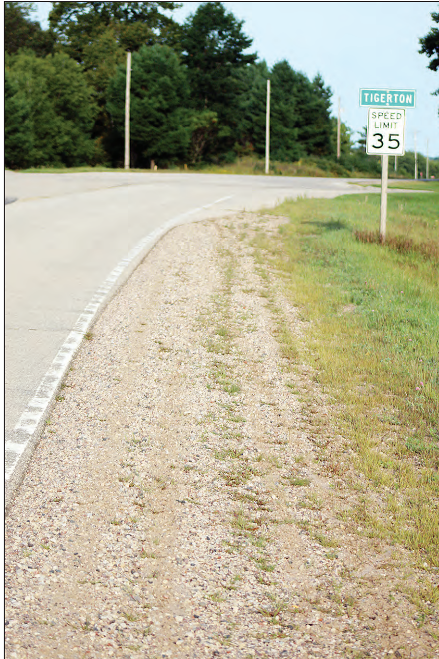
A portion of County Road M near Tigerton was designated as an off-highway motorcycle route by Shawano County.
