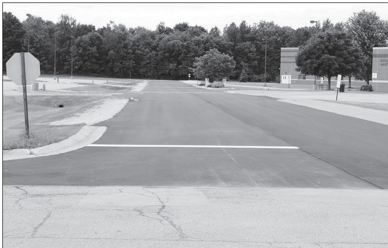
Work was recently completed on one of the access roads in the Shawano Community High School parking lot.
