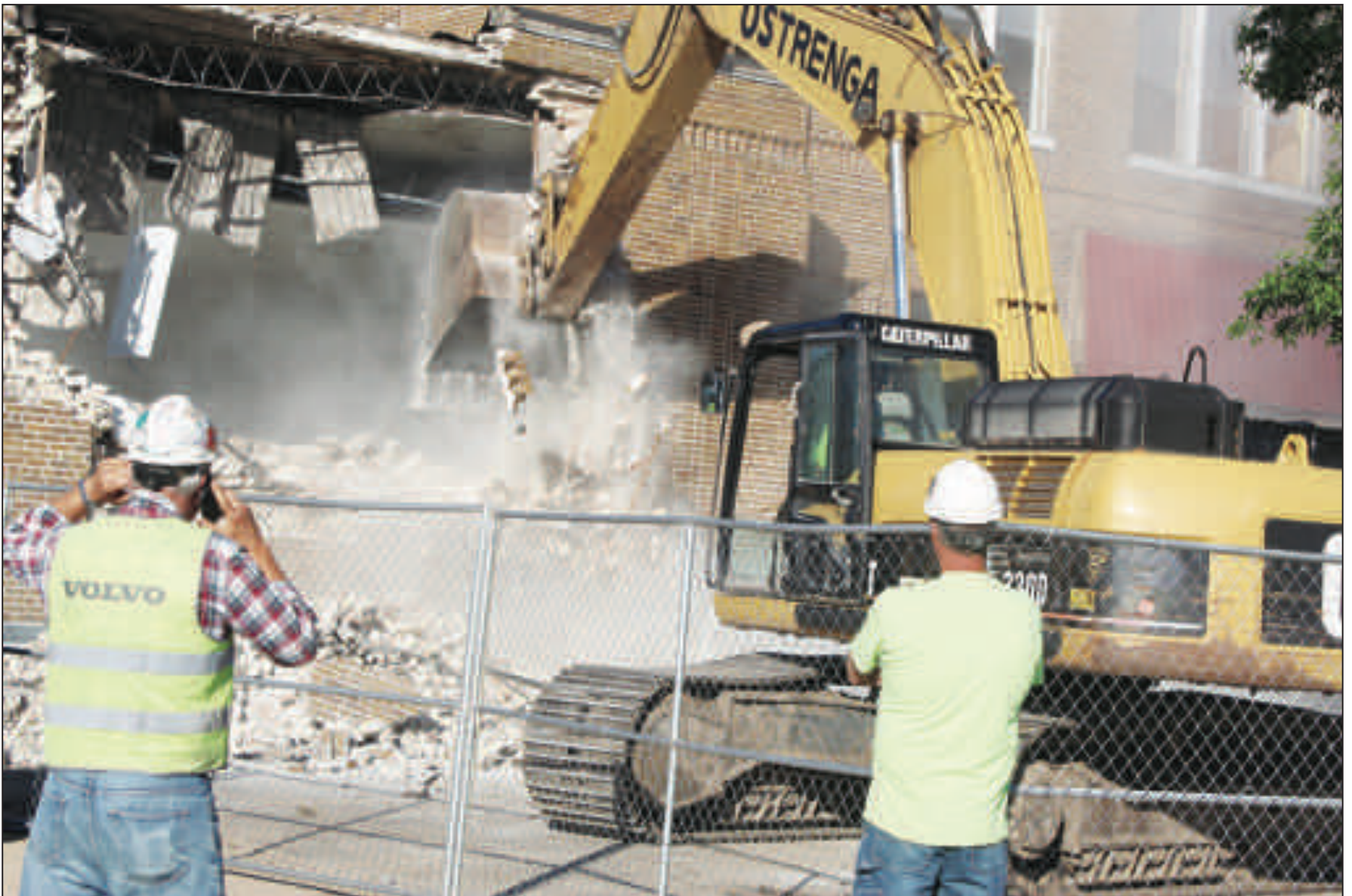
A portion of the original Gresham Community School built in 1935 is demolished Tuesday morning in preparation for the second phase of a renovation project approved by voters in 2018. The school's new cafeteria, offices and additional classrooms will go where the old school used to be.
