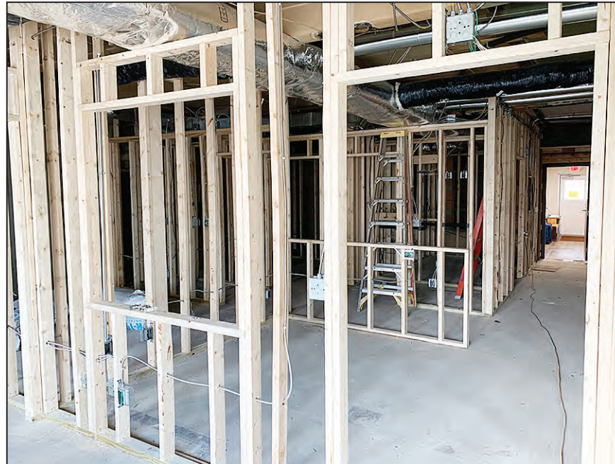
A free health care clinic is in the process of being built at the SAM25 shelter on 105 E. Richmond St. in Shawano. The health care clinic will service those who cannot afford health insurance.
