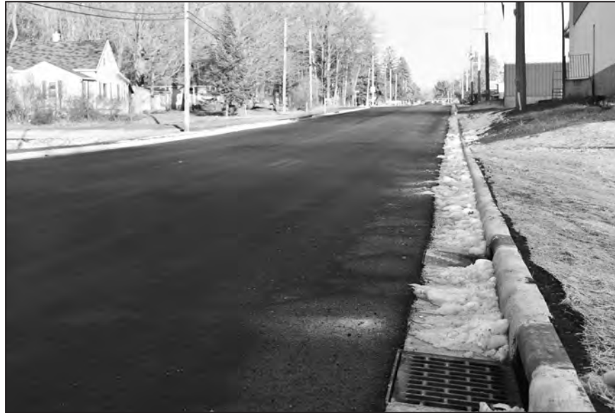
This year's construction project rebuilt Washington Street in Gillett from a rural road into an urban street with curb, gutter, water main and storm sewers.
