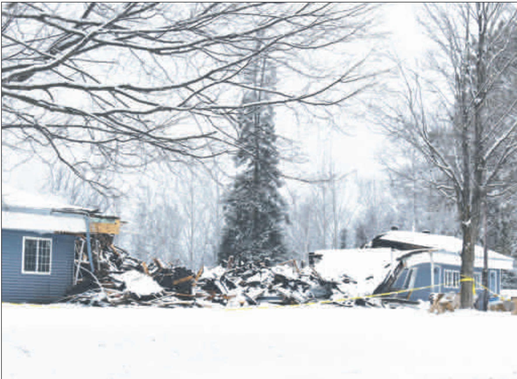
The restaurant portion of the Golden Eagle building, which was called the Red Arrow Motel when it opened in the 1950s, was leveled in the Dec. 18 blaze. The structure is considered a total loss.
