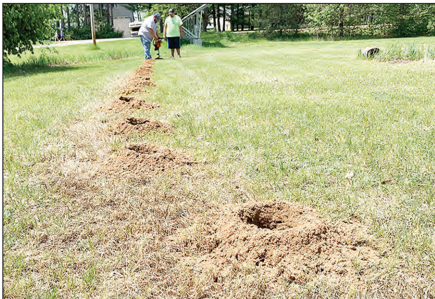
Menikanaehkem executive director Anahkwet “Guy” Reiter begins the preparation of building the lodge by digging holes at the Menikanaehkem complex on May 22.
