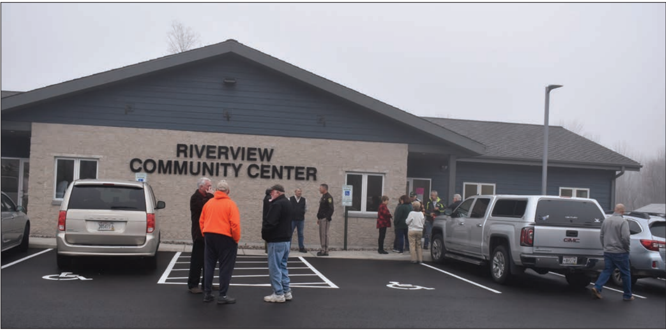
Dozens of local residents take advantage of the opportunity to tour the new Riverview Community Center during an open house Nov. 16.
