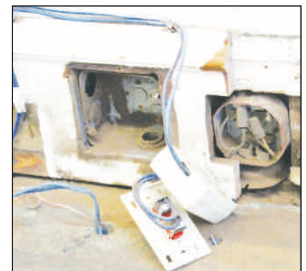
One example of the electrical nightmare addressed in the recent upgrade was the discovery of live wires that once powered the X-ray machinery of the now-defunct hospital. The electrical upgrade led to a much bigger restoration of the building that now hosts the ThedaCare clinic in Tigerton.
