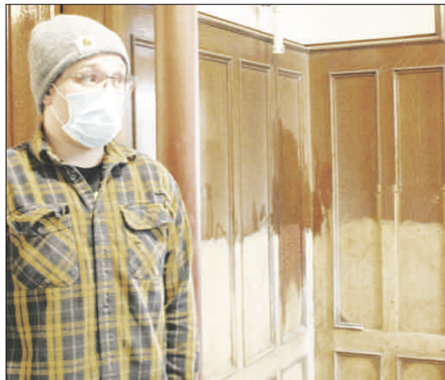
Aaron Damrau pauses in his restoration work at the Swanke mansion in Tigerton. He's standing near some of the oak woodwork in the entryway that's being refinished. Herman Swanke used generously the wood and millwork produced in his Tigerton Lumber Company in building the home in 1920.
