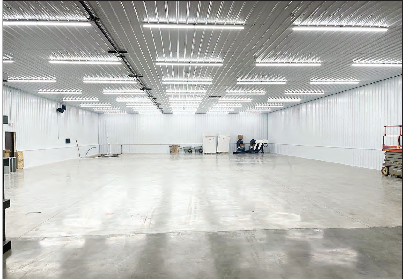
The new expansion for JR Machine in Shawano is expected to be ready by early April.
