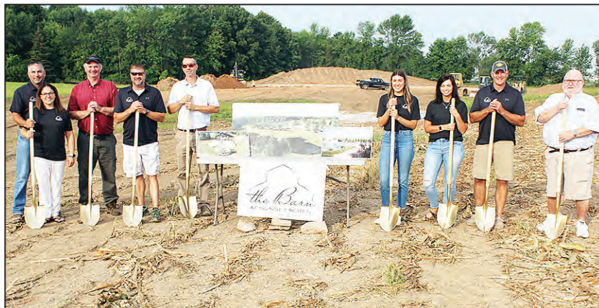
The official groundbreaking for the Barn at Sunset Acres on the north side of Pulaski took place Aug. 23, but in the background, heavy equipment is already flattening the area so building can begin and hopefully be complete by summer 2022.
